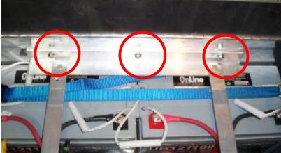
**Step 3**: *Right;* Fold the shelf support as shown and remove. Be careful that it does not touch the battery terminals and cause a short-circuit.
